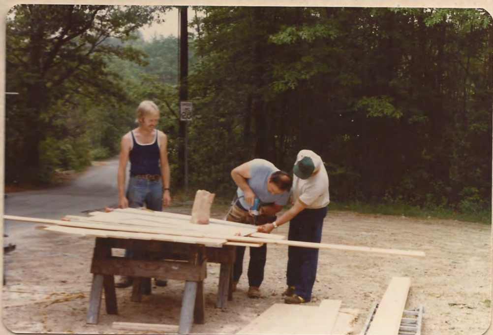
1981 Building shutters for the club.
